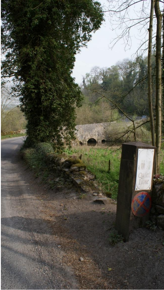
c) Approaching Conksbury bridge from the south
